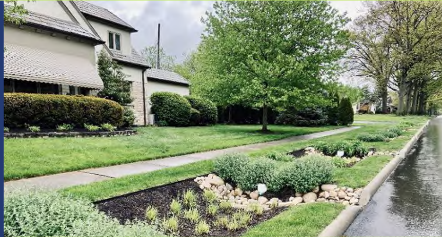
Behind-the-curb rain garden- no walls
