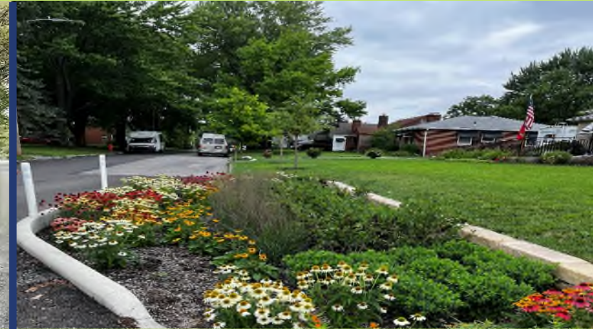
Bump-out rain garden
