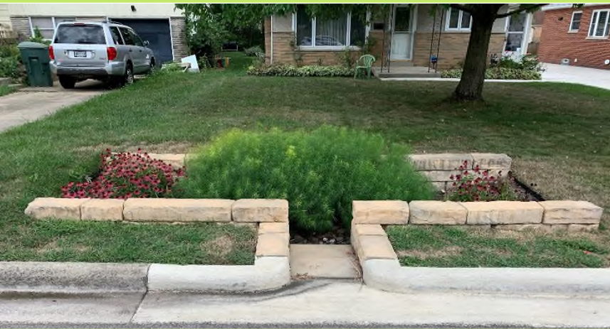
Behind-the-curb rain garden- 2 walls
